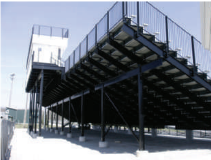
Column and Beam
