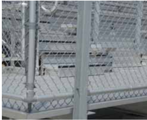
Galvanized Chain Link Fence
