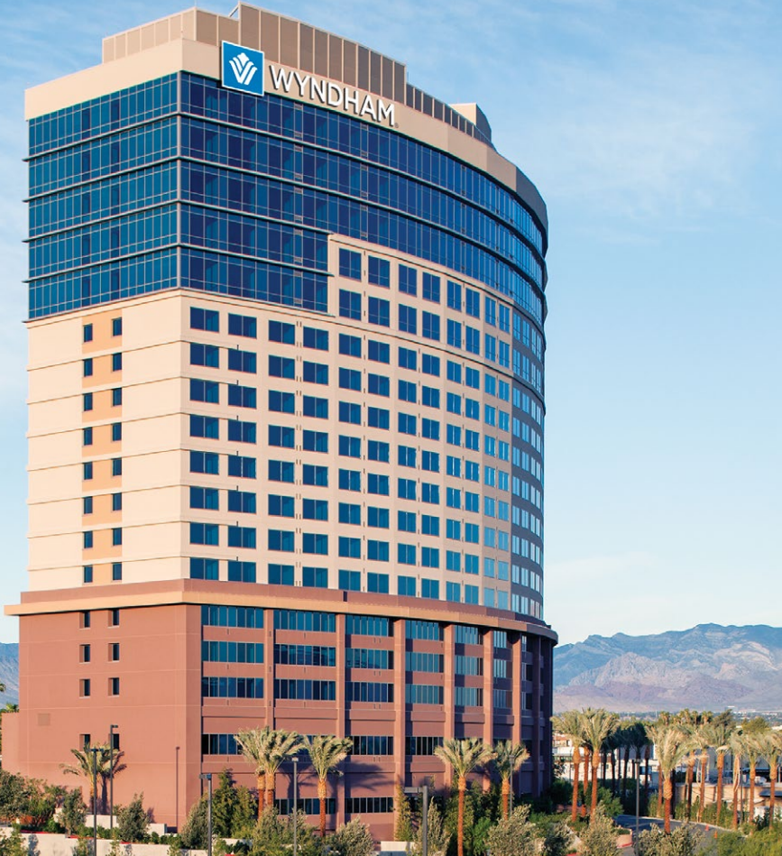
WYNDHAM DESERT BLUE | Location: Las Vegas | Products: Pacifica ® Glass, Solarban ® z50 Glass Architect: KGA Architecture | General Contractor: Martin-Harris Construction Glass Fabricator: Oldcastle BuildingEnvelope® | Glazing Contractor: Walters & Wolf Photo courtesy of Tom Kessler Photography
