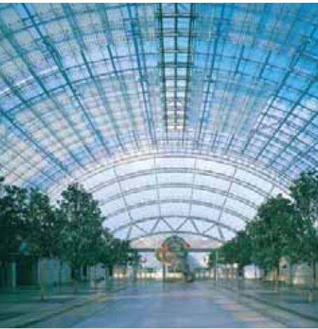
▲ Leipziger Messe Neues Messegelände Location: Leipzig, Germany Products: Starphire ® Ultra-Clear Glass Architect: Von Gerkan, Marg & Partner Glazing Contractor: Ian Ritchie Architects
