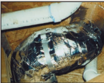
Contours easily to elbows that are required in maximum 20 ft. ducts.
