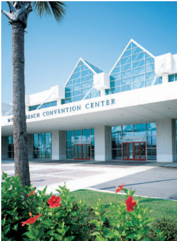
Myrtle Beach Convention Center, Myrtle Beach, SC Architects: Cannon Associates
