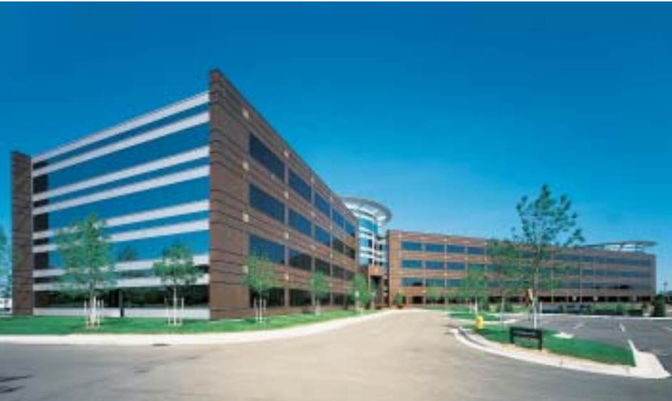
below: Corporate Crossing Dearborn, MI Neumann Smith & Associates CW-600 with granite & aluminum panel infill
