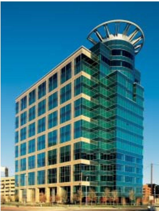
left: Millenium I Dallas TX HKS Architects CW-600 with glass and granite
