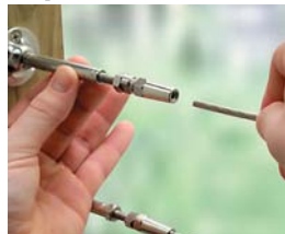
Fully seat wire rope.
