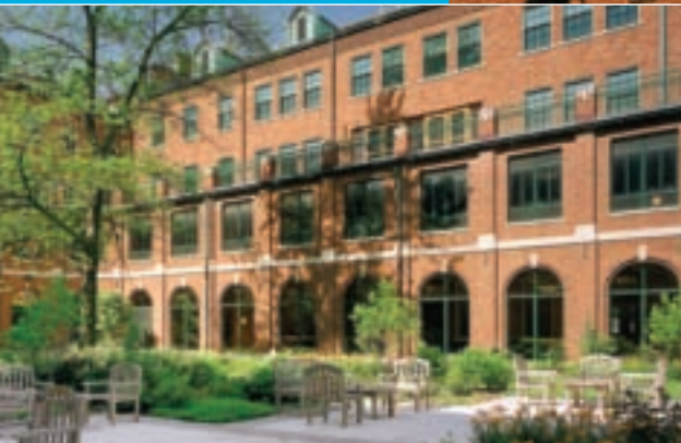
Immaculate Heart of Mary Mother House Monroe, MI Architect: Susan Maxman and Partners
