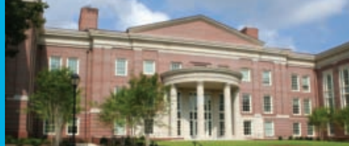
University of Georgia-Coverdale Center Athens, GA Architect: HOK
