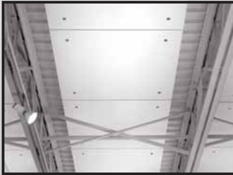
Optima Capz, installed 2-3/4" from a metal deck.
