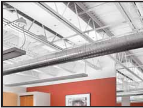
Optima Capz, installed 6-1/2" from a metal deck.
