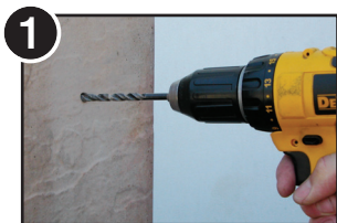
1 Drill 1/4" hole with masonry bit to 1-1/2" (minimum) depth. Blow debris out of hole.
