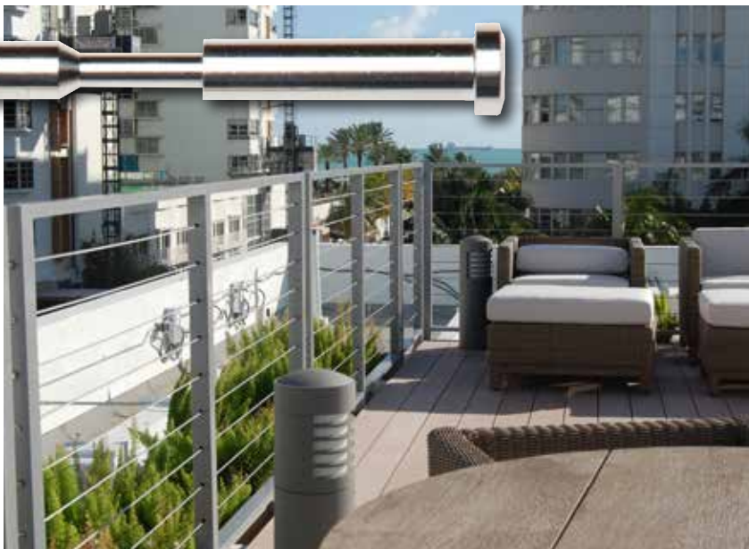
The Redbury South Beach - Miami, FL Rail Fabricator: Climatrol Quality Aluminum Cable Supplier: Sailing Services, Inc. - Miami, FL
