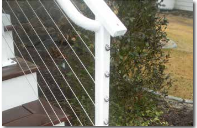
Private Home - Old Lyme, CT Cable Fabricator: OCD Rigging - Chester, CT
