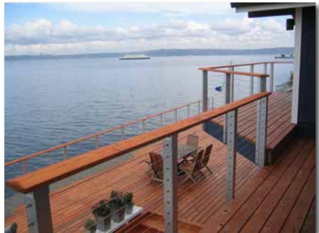
Private Home - Tacoma, WA Cable Fabricator: American Metal Specialties - Tacoma, WA
