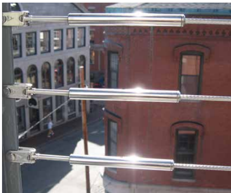
Portland Regency Hotel - Portland, ME Cable Fabricator: NE Tech Air & Maine Steel - Scarborough, ME
