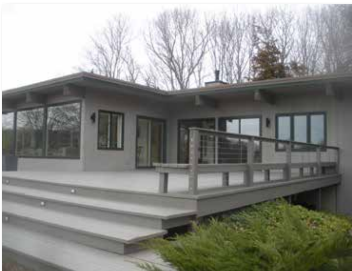
Private Home - Old Lyme, CT Cable Fabricator: OCD Rigging - Chester, CT
