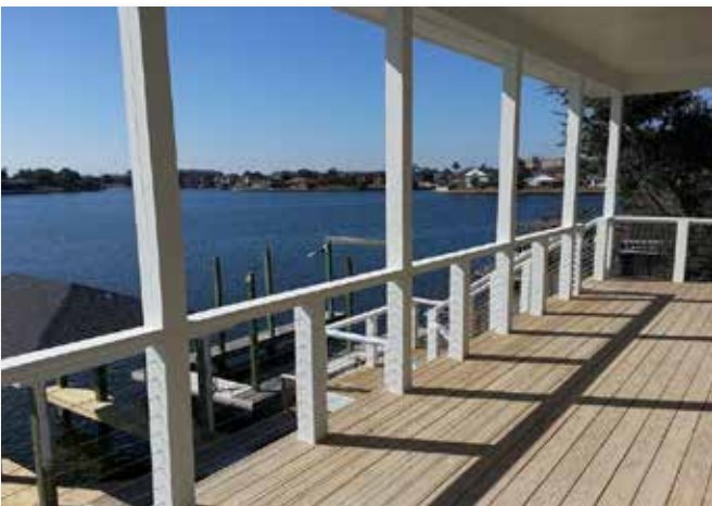
Private Home - Galveston, TX Cable Fabricator: Bahama Rigging - Kemah, TX
