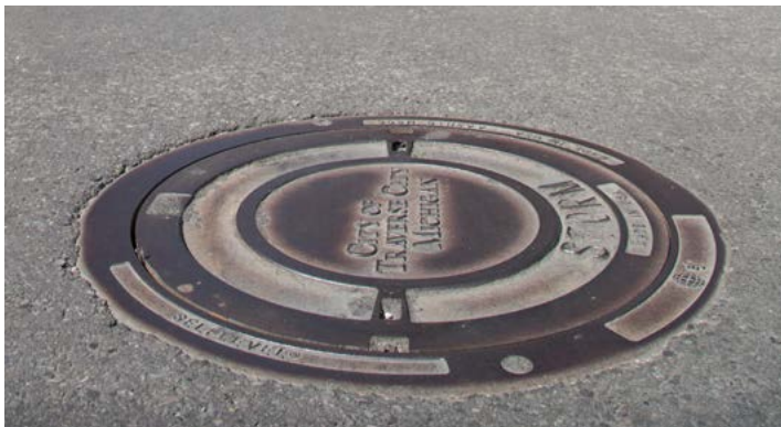
SELFLEVEL installed in Traverse City, Michigan.
