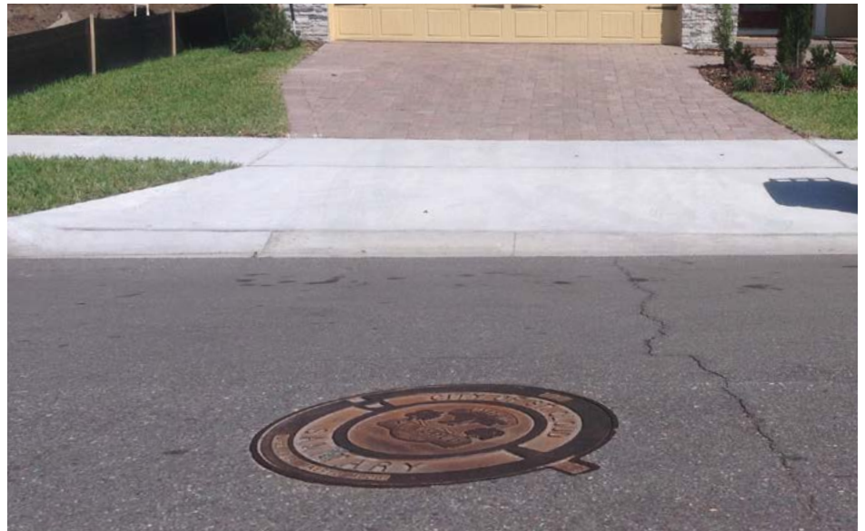
ERGO access assembly in the City of St. Cloud, FL.
