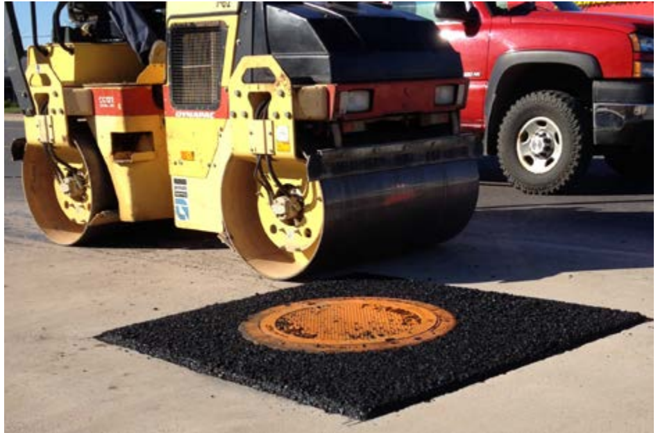
After asphalt has been packed, the SELFLEVEL compacts level with the surrounding roadway for a smooth finish that will last longer than traditional manhole assemblies in situations where there can be frost heave and natural road settling.
