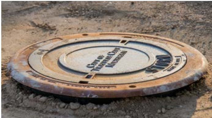
With backfill packed around the guide frame, this SELFLEVEL is prepared for asphalt at a new installation in Traverse City, Michigan.
