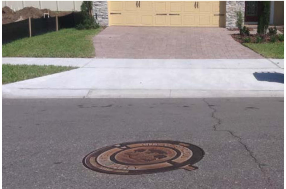
ERGO access assembly in the City of St. Cloud, FL.
