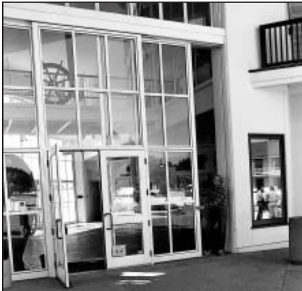
#974 Steel Plate Sliding Doors Maritime Museum, Monterey, CA
