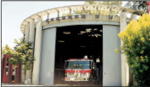
Berkely CA Fire Station 4 Panel Curved Telescoping, Sliding Electronically Operated 24'x17' Doors
