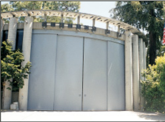
Electrically operated sliding curved door Berkley Fire Station, Berkley, CA
