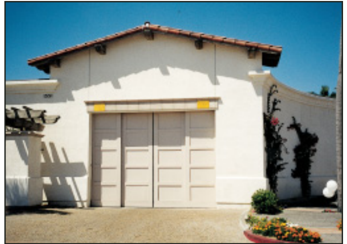
Electrically operated telescoping doors Kona Kai Hotel, San Diego, CA
