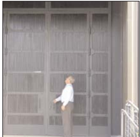
DiRosa Art Preserve, Napa, CA #948 Steel Frame Door with Tongue and Groove Redwood Strips.
