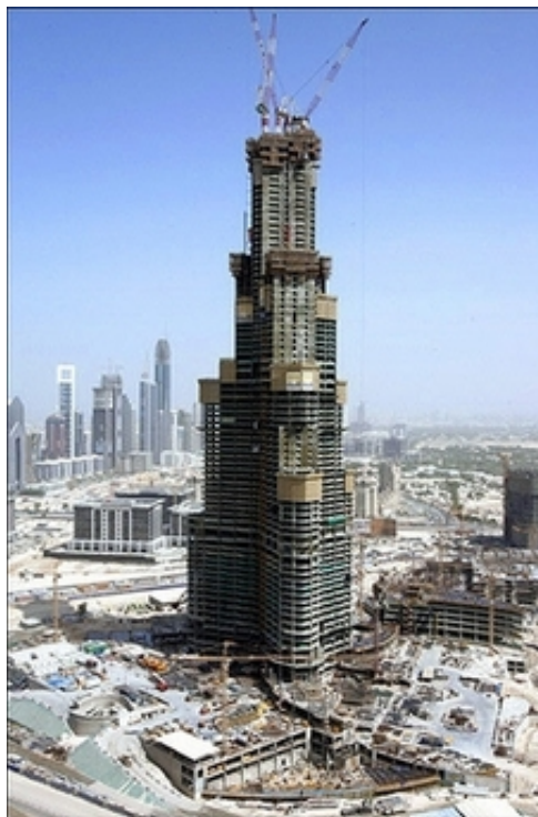
Delivery of most Culligan equipment to the Dubai Tower is expected to take place in 2007.
