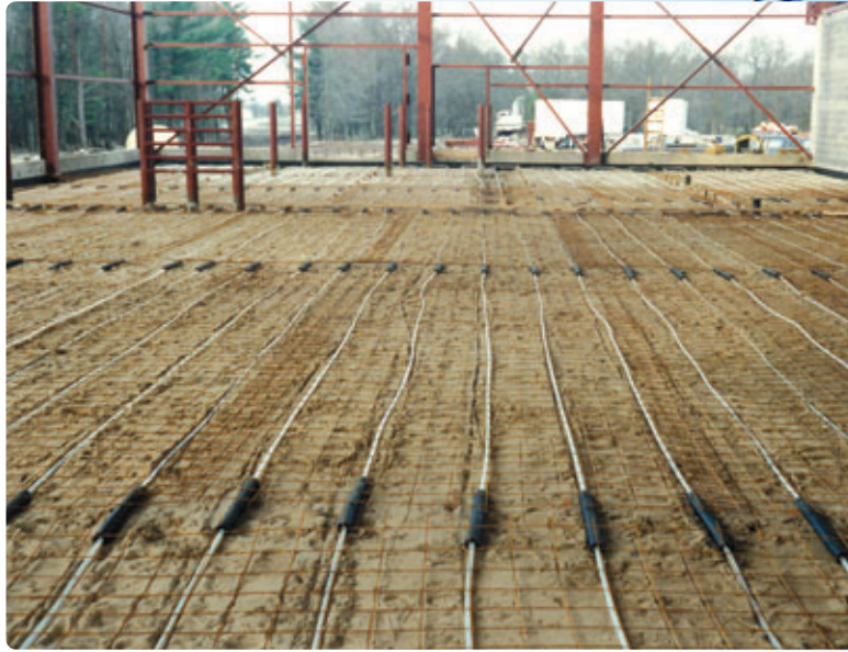
PEX tubing ready for backfill covering in a new cold storage facility
