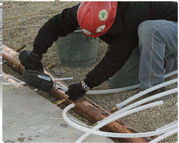
A contractor uses an expander tool to make an Uponor ProPEX® fitting during the installation of a turf conditioning system at a professional soccer team's new stadium (Chicago Fire).
