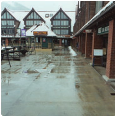
Operation photo from a ski resort in Park City, Utah
