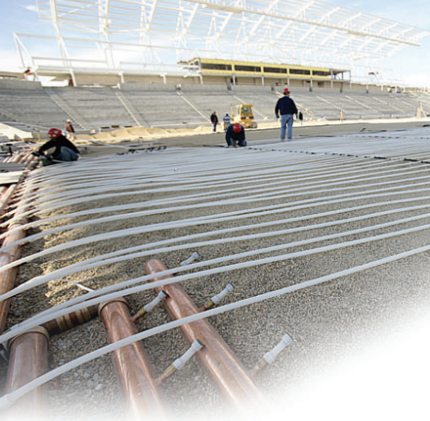
A contractor uses an expander tool to make an Uponor ProPEX® fitting during the installation of a turf conditioning system at a professional soccer team's new stadium (Chicago Fire).
