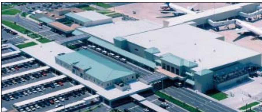
Orlando/Sanford Airport Orlando, FL
