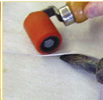
Fig 2: The Seam – Triple welded, 1½" seam
