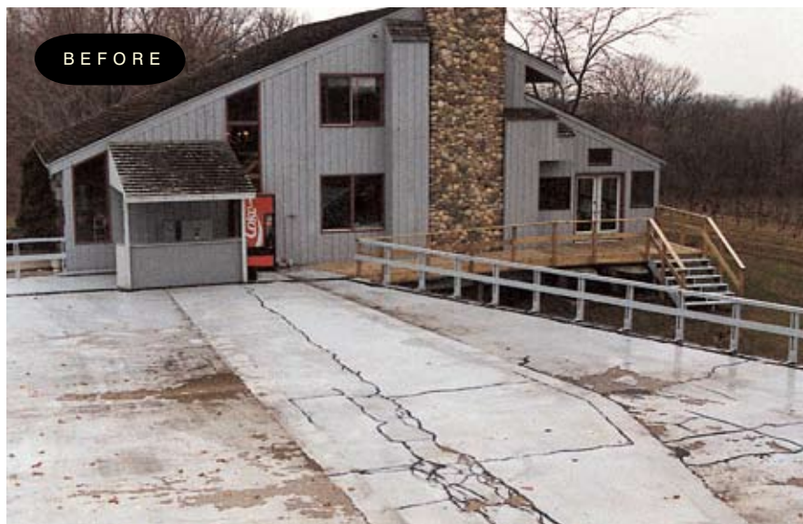
LEAKING, UNSIGHTLY ROOF OVER WINERY
