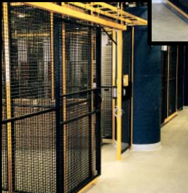
Dual-Color Powder Coated Co-location Cages @ network information hub
