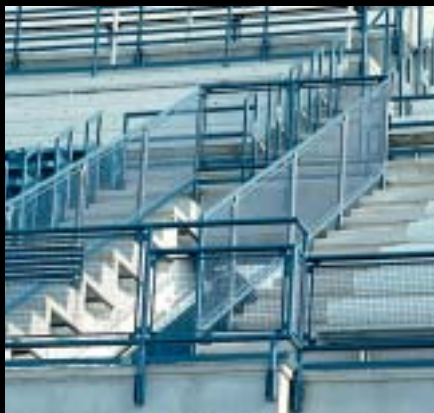
Railing Infill Panels Fitzgerald Tennis Center, Washington, D.C.
