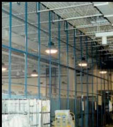
Registry Cage Bulk Mail Facility, Washington, D.C.
