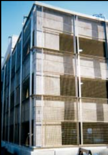
Bronze Anodized Façade Grilles J.B. Speed Art Museum Parking Garage Louisville, KY
