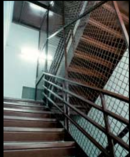
Stairway Partitions First Union Tower Baltimore, MD
