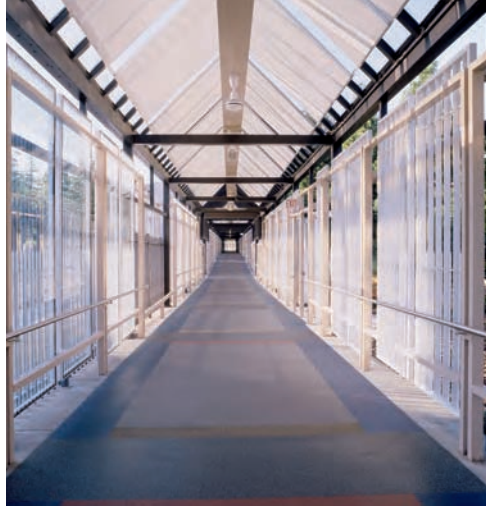
ECOearth, Duke University Medical Center walking bridge, NC Architect: Duda Paine Assoc. Honorable mention, 2005 StarNet® Design Awards
