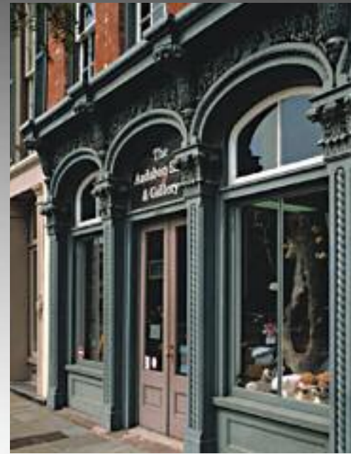
Meeting Street Restoration Charleston, South Carolina
