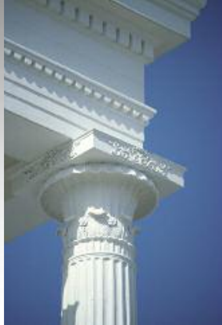
Alabama State Capitol Montgomery, Alabama Monumental Greek Revival column capitals are faithful reproductions of the originals cast in the 1850s. Six feet in height with an abacus seven feet square, each capital weighs approximately one ton.
