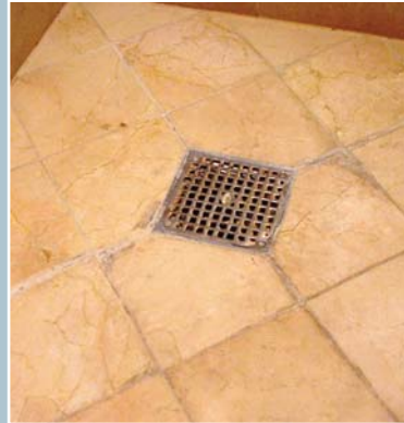
Tiled shower floors can leak and have mold problems
