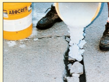
Abocrete fills voids and replaces missing sections of concrete.
