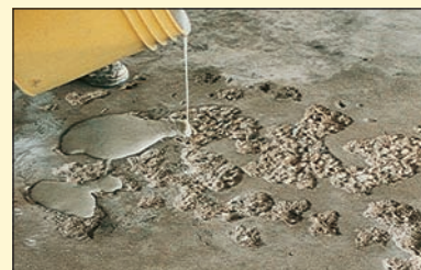
Abocrete repairs spalled concrete.
