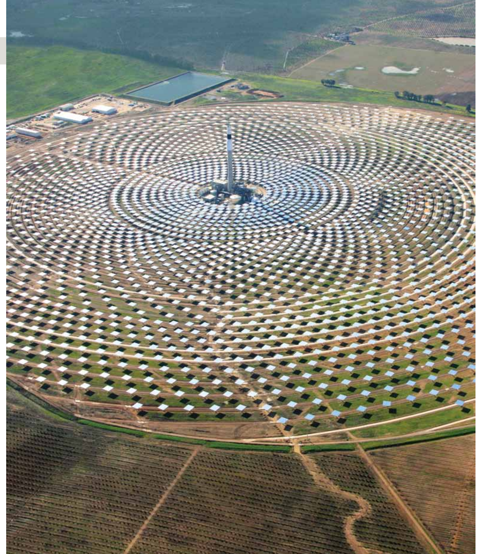
EcoGuard flat laminated mirrors were used to create Gemasolar, a solar energy plant distinguished by its ability to generate high power outputs in the absence of solar radiation.
