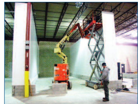
Steel Reinforced Tied to Building Structure
