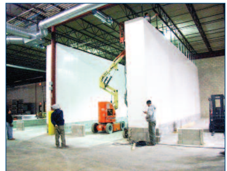
17 Foot High Panels on 2 Foot Block Wall
