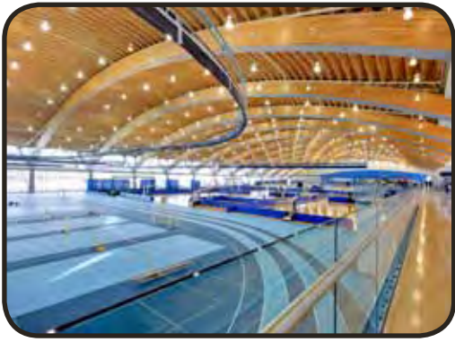
Robbins All-Star™ Portable and Pulastic System Richmond Olympic Oval Installed by: Centaur Products
