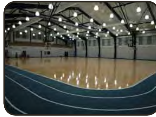
Robbins Sportwood Ultra Star and Pulastic® Fusion System Copley High School Installed by: Cincinnati Floor Company
