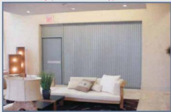
when activated the Safescape® S9000 creates both the fire & smoke protection necessary while also allowing for Emergency Egress.
