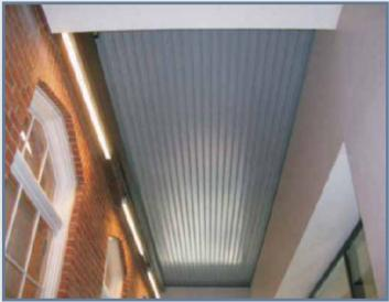
Horizontal coiling fire shutters for protection of openings in ceilings
