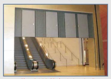
When activated, the fail-safe system lowers the coiling fire curtain and swinging emergency egress doors down into position....
