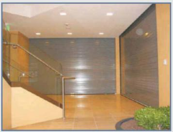
Temperature rise rated fire doors are required when used in exit enclosures or exit passageways
