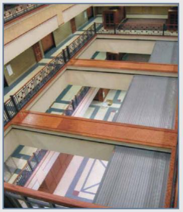
H200 horizontal coiling fire & smoke shutters used in an atrium application
