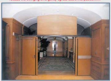
Within seconds, the fail-safe fire door system lowers the coiling fire curtain into position without the aid of any electricity or battery back-up system.....
