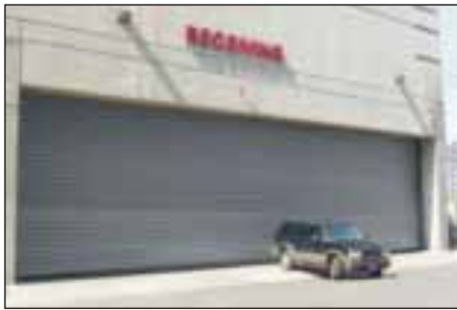
70 Foot wide Hurricane Door provides the necessary protection without limiting daily business operations
