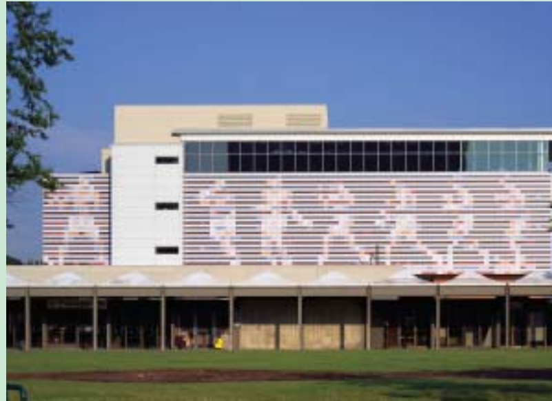
Muhammad Ali Center in Louisville, KY. Custom-colored KerAion Quadro façade panels form silhouettes.
