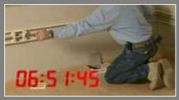
After inserting dividers, wires are pulled, wire clips added, and receptacles are wired up and installed. After more measuring and cutting, covers are installed.
