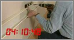
The electrician has to measure, cut, and install base sections individually.
