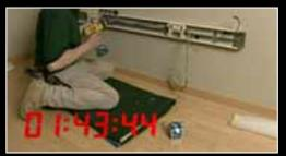
The electrician simply installs prewired sections. There's no measuring, no cutting, no wire clips, and no wiring up individual receptacles.
