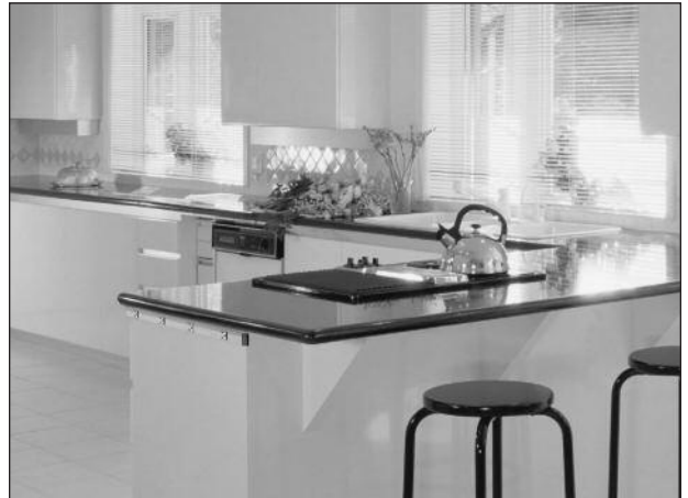
2000 Series Plugmold installed in a residential kitchen.
