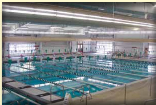
Westside Aquatic Center Gutter Evacuator™ Install Greenville, SC
