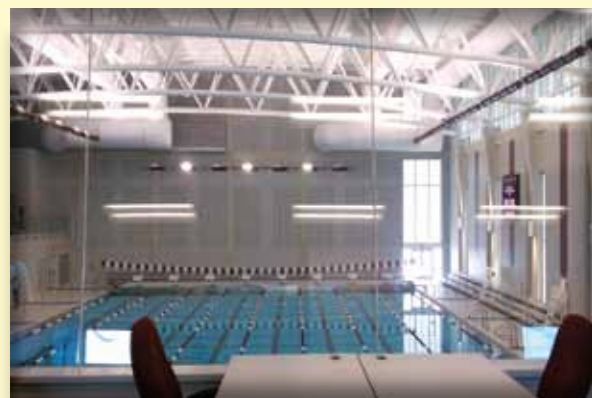
Jenks Aquatic Center Gutter Evacuator™ Install Jenks, OK
