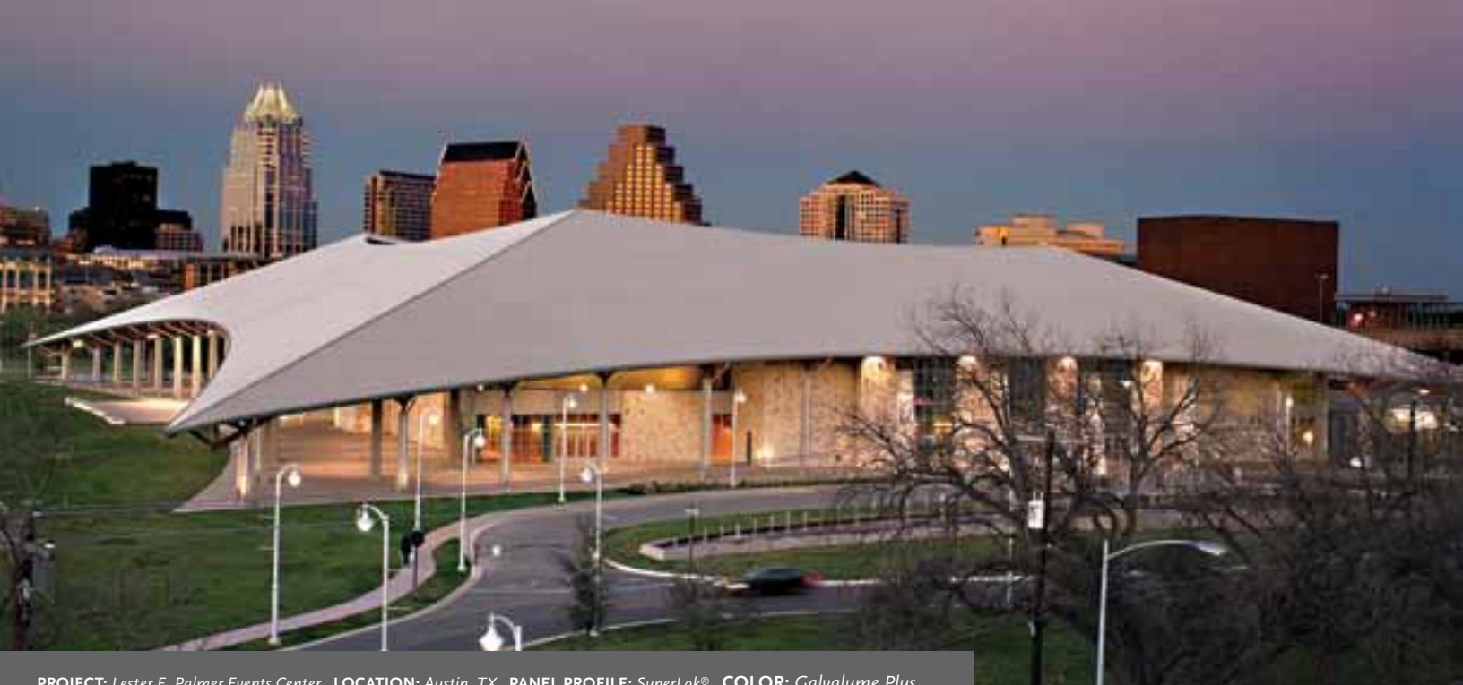
PROJECT: Lester E. Palmer Events Center LOCATION: Austin, TX PANEL PROFILE: SuperLok® COLOR: Galvalume Plus
