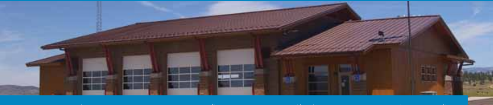
C PROJECT: UDOT Strawberry Maintenance Station LOCATION: West Valley, UT PANEL PROFILE: Double-Lok® & Artisan® Series COLOR: Champagne Metallic
