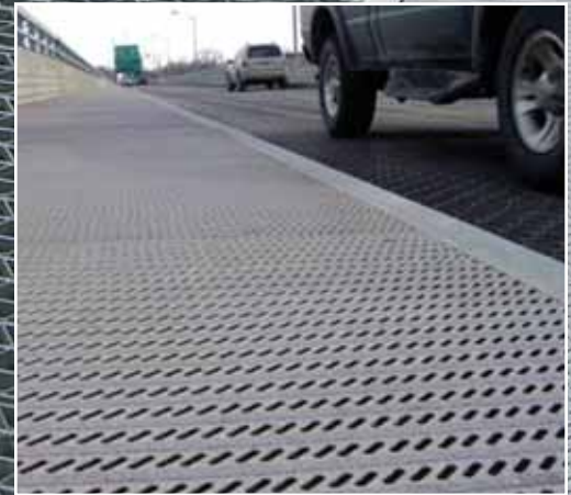
Grosse Ile Bridge, MI - Aluminum Plank Walkway
