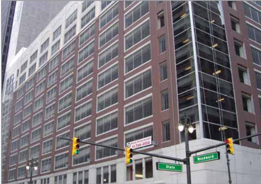
▲ Woodward Parking Garage - Detroit, MI
