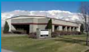
INTERSTATE GRATINGS, UT ▲
