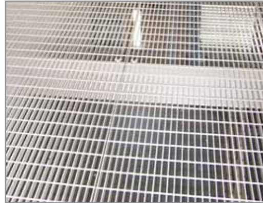
◀ Detail -North Carolina State Feed Mill - Raleigh, NC
