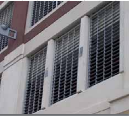
▲ Woodward Parking Garage (typical 4 x 12 infill detail)
