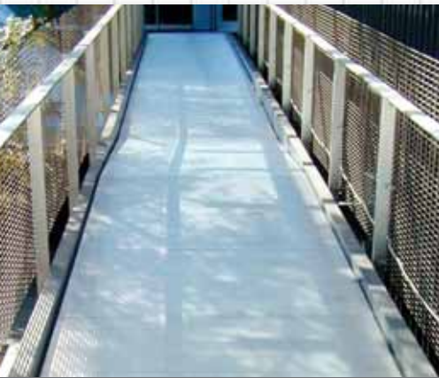
Pedestrian Bridge ▲ (7-SGi-4) Corning, NY
