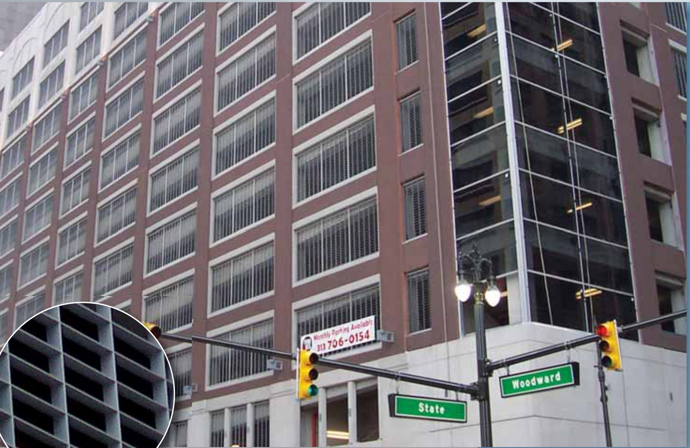
▲ Woodward Parking Garage Grille - Detroit, MI (4 x 12 infill)
