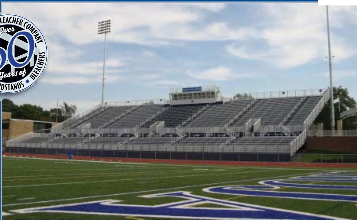
CHAMBERSBURG, PA - 38 row by 210' football stadium that seats 4,420. IL2K decking system. Vertical Rail and a 8' by 42' sloped front pressbox. Designed by Crabtree Rohrbaugh & Associates. Manufactured and installed by Southern Bleacher.
