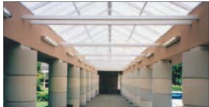
ID 3147 – Andover High School, MI O.E.M. Architects, Inc. Pre-engineered ridge walkway cover enabled efficient installation of school walkway.
