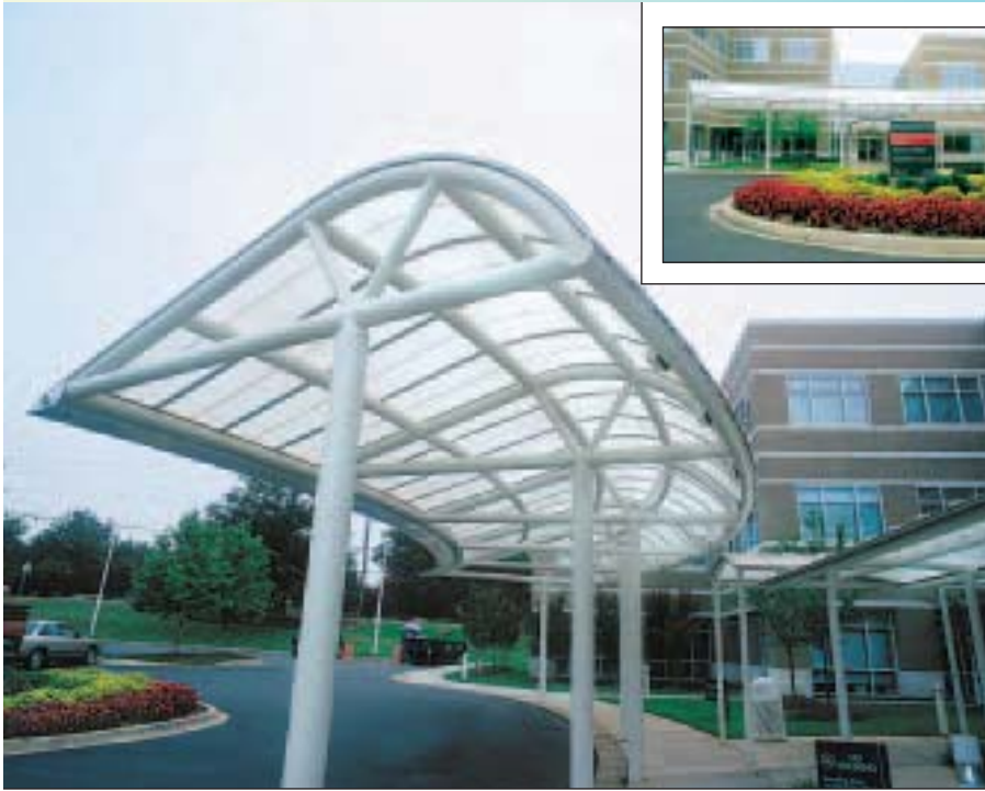
ID 3495 - Greenville Hospital, Greenville, SC
