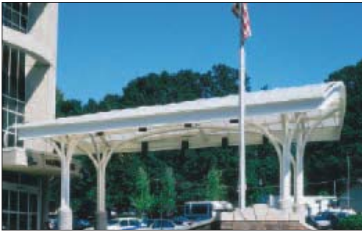
ID 1099 – St. John's Home, NY Blakeheld-The Dewolff Partnership Architects Dualwall® skinned over round tube structure for visually interesting entrance.
