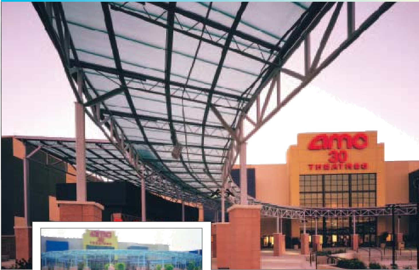
ID 1276 – AMC 30 Theatres, TX Gould Evans Goodman Assoc. Architects Green Dualwall® skinned over a steel structure for economy and exciting appearance.
