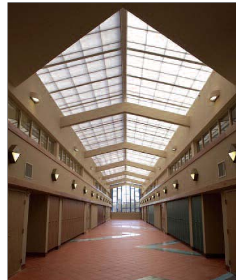
ID 9036 - American Hebrew Academy, Greensborough, NC Skylight with Class A Roof Construction configuration Architect: Aaron G Green Associates, San Francisco, CA
