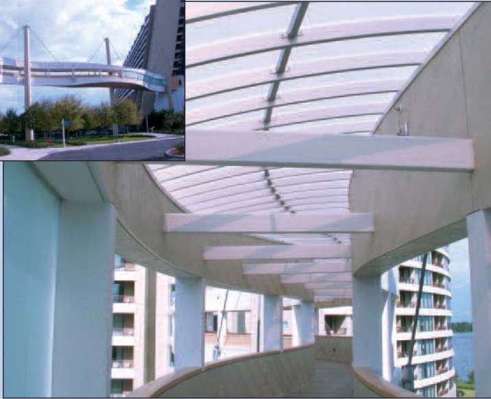
ID 28138 - Translucent Walkway Cover for an amusement park, Orlando, FL Architects: Gwathmey Siegel & Associates, New York, NY; Glover-Smith-Bode, Inc., Oklahoma City, OK CPI used U-Lite™ to construct this self-supporting aluminum skylight. This challenging project links old and new hotels with a winding walkway.
