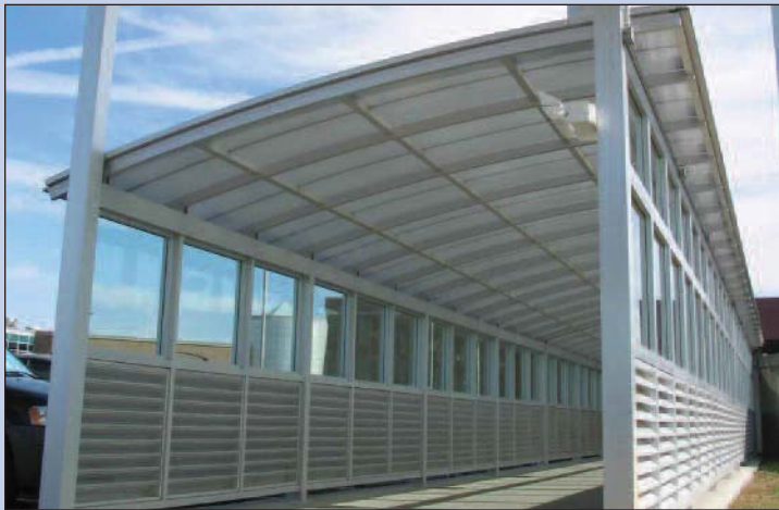
ID 15987 - Amarillo Airport, Amarillo, TX Architect: Reynolds, Smith and Hills Inc, Jacksonville, FL CPI provided the entire system from the ground up.
