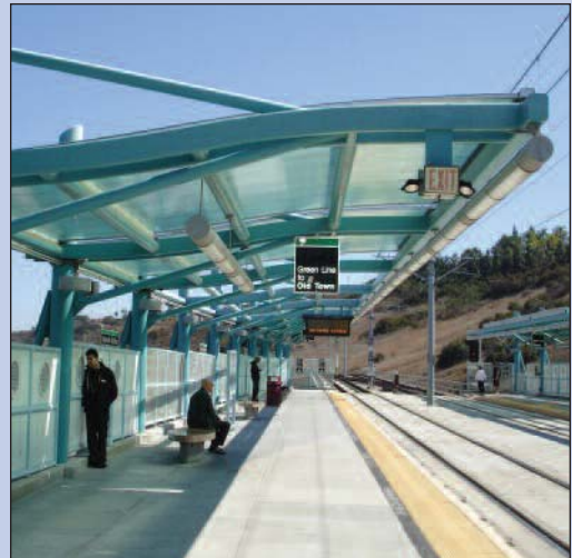
ID 13279 - Mission Valley East Light Rail Station, San Diego, CA Architect: Parson Architects This light rail drop-off canopy consists of 9,000 SF of Pentaglas® 12.
