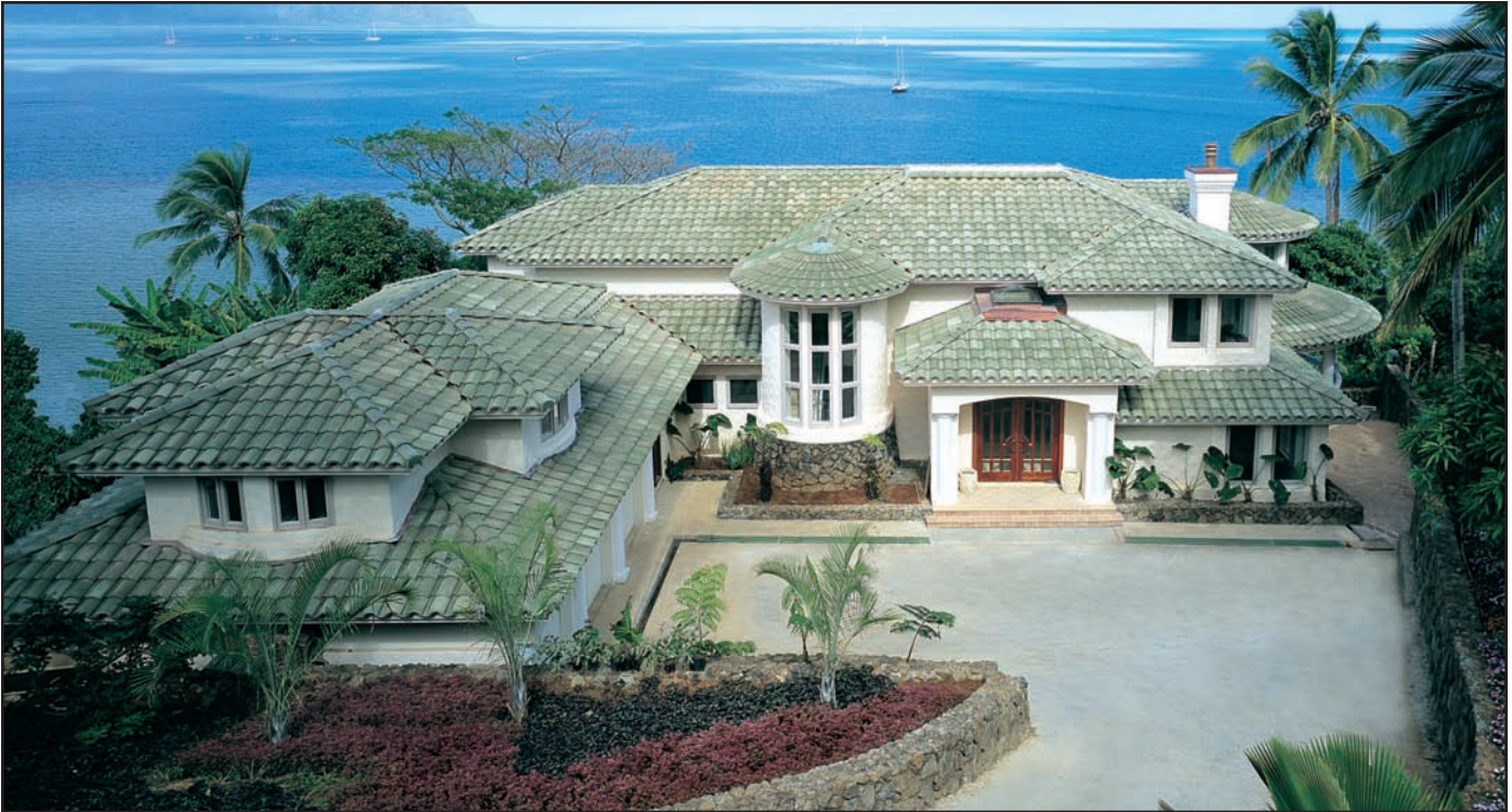
Kaneohe Bay, Hawaii Custom House - Weathered Green Blend 305 Straight Barrel Mission with various sizes of Turret Tile™
