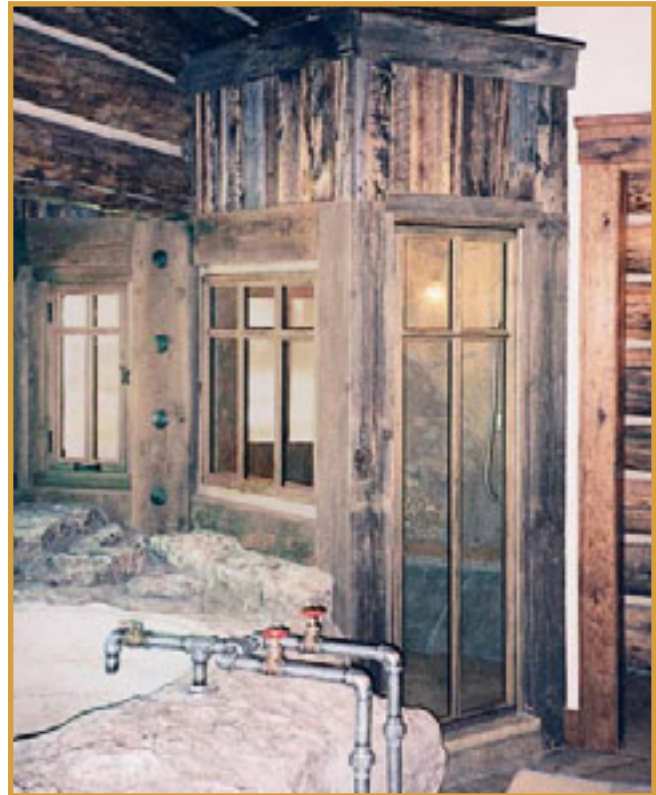
▲ Yes, it is a wood overlay on a shower door. Black powder coated metal is used on the interior of the unit for durability in the shower.
