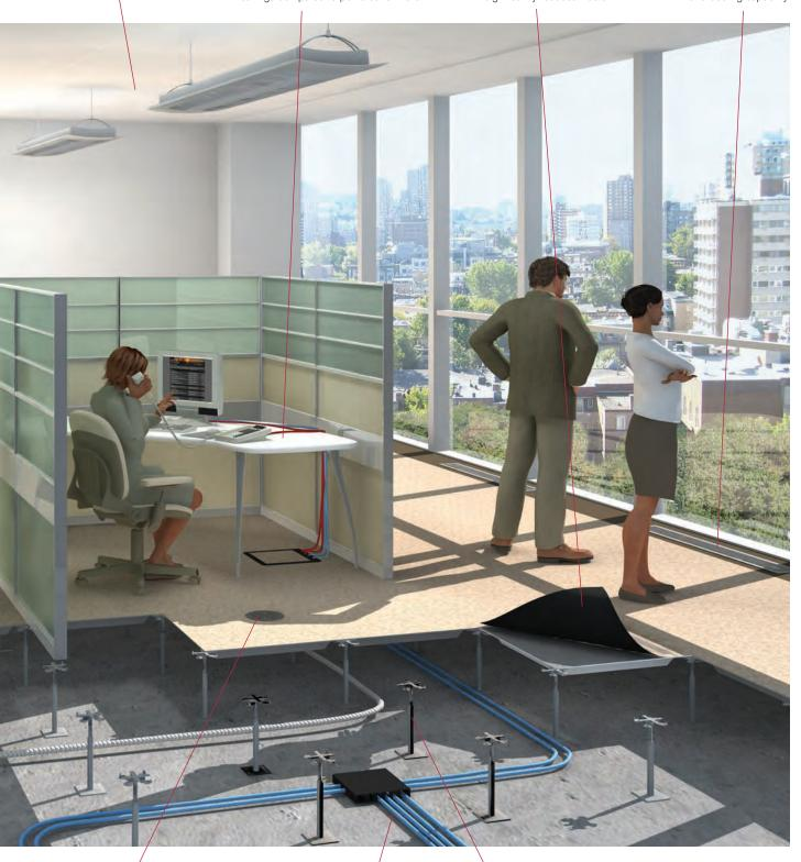
Underfloor service pathway accommodates any type of voice and data system approach, from homerun to passive or active zone cabling
