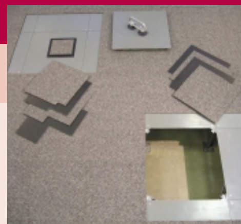
Step 2: Remove four cut carpet tiles from around service box...
