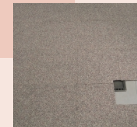
Step 6: Cut carpet tiles do not fit at new location, need new carpet tiles...
