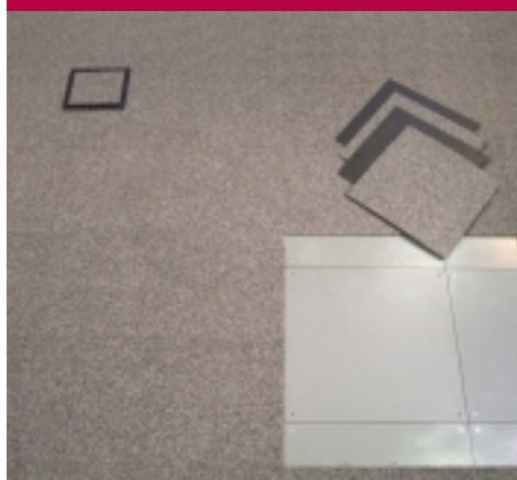
Step 1: Remove four 18"x18" carpet tiles to expose one panel...
