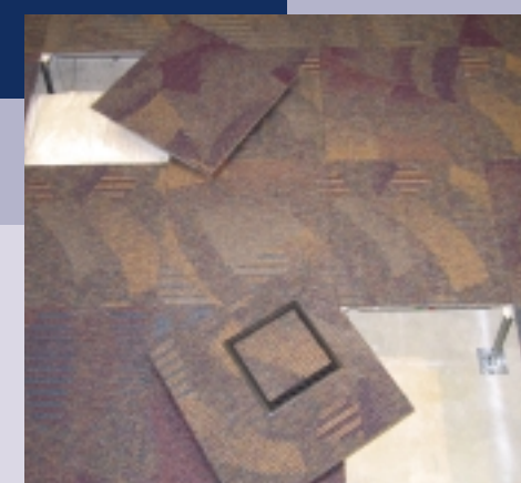
Step 3: Switch the service panel with the solid panel...
