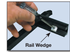
Tightening rail wedge on shortened section.
