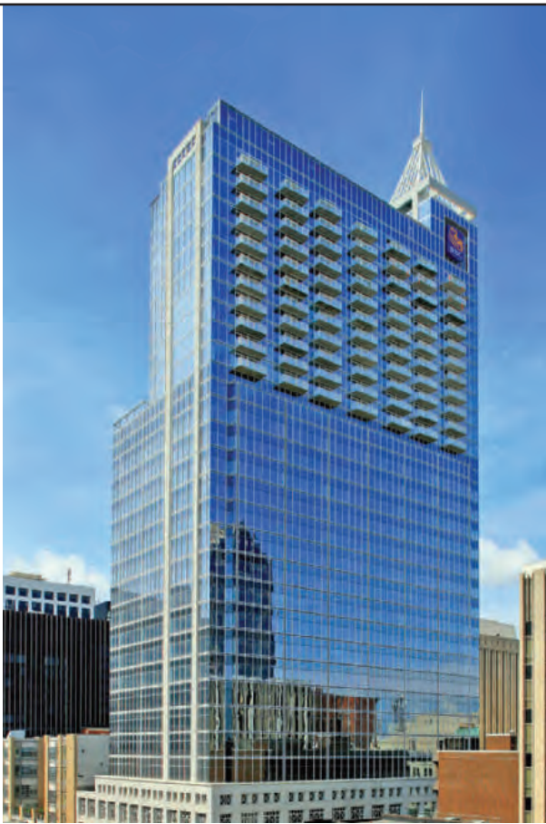
RBC Tower, Raleigh, North Carolina Architect: Cooper Carry Glazing Contractor: Harris/Carter Wall Systems Systems Used: YCW 750 OG, YCW 750 IG, YCW 250, YWW 50 T with slab edge cover, YSD 400, & Model 35D
