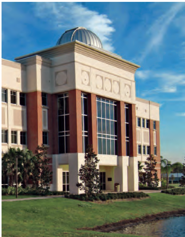
FW: Olin Physical Science Building, Florida Institute of Technology, Melbourne, Florida Architect: STH Architectural Group, Inc., Glazing Contractor: Miller Glass & Glazing Inc., Systems Used: YHC 300, YHS 50, & Model 35H
