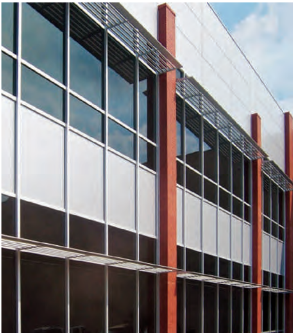
Brick Street mutual Insurance Co., Charleston, West Virginia Architect: Associated Architects, Inc. Glazing Contractor: Central Glass of Charleston Systems Used: ThermoShade™ & YCW 750 OG
