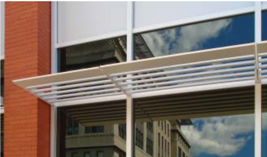
Brick Street Development, Charleston, West Virginia Architect: Associated Architects, Inc. Glazing Contractor: Central Glass of Charleston Systems Used: ThermaShade™ & YCW 750 OG
