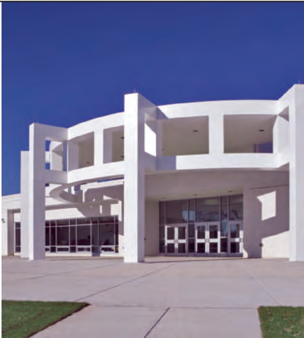
School of the Future, Philadelphia, Pennsylvania Architect: The Prisco Group Glazing Contractor: US Glass and Metal Systems Used: YCW 750 OG, ThermaShade™, & Model 50D LEED Gold Certified
