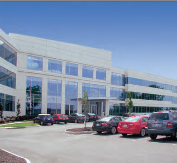
BMW Automotive, Columbus, Ohio Architect: URS Glazing Contractor: Anderson Aluminum Systems Used: YCW 750, & YWW 45 TU
