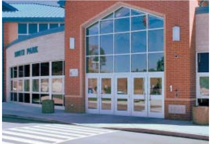
South Park High School, South Park, Pennsylvania Architect: Foreman Architects Glazing Contractor: Specified Systems, Inc. Systems Used: YCW 750 OG, YES 45 TU, YOW 250 T & 50D
