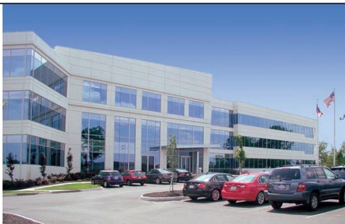
BMW Automotive, Columbus, Ohio Architect: URS Glazing Contractor: Anderson Aluminum Systems Used: YCW 750, & YWW 45 TU
